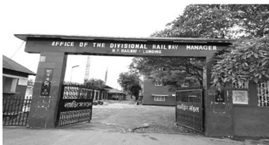
Lumding Railway Station
