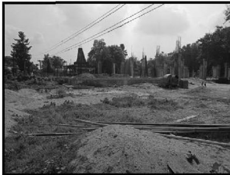
Ongoing construction of Modern Town Hall at Rangapara Town
