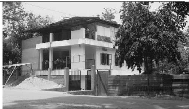
A Pucca house with typical structure
